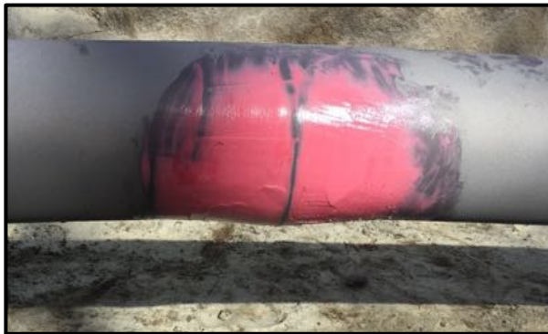
High compressive modulus load transfer epoxy used to smooth anomaly
