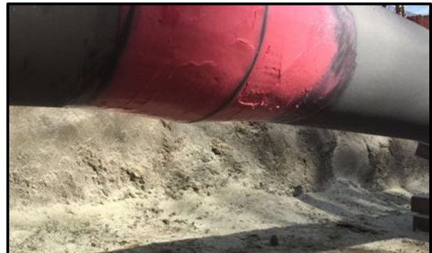
High compressive modulus load transfer epoxy used to smooth anomaly
