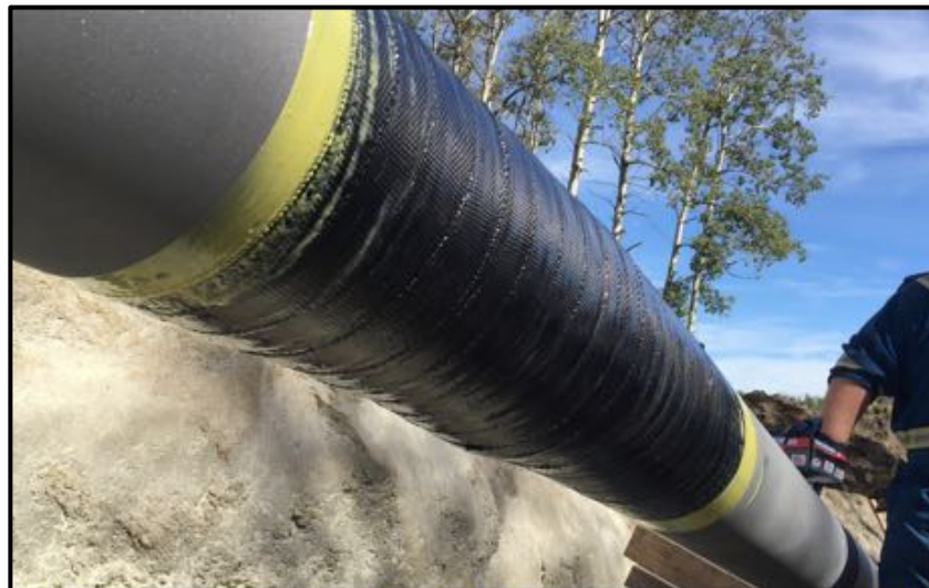
Completed DiamondWrap® HP™ repair
